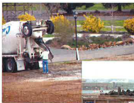
Figure 1. Chute washwater being dumped on the ground
