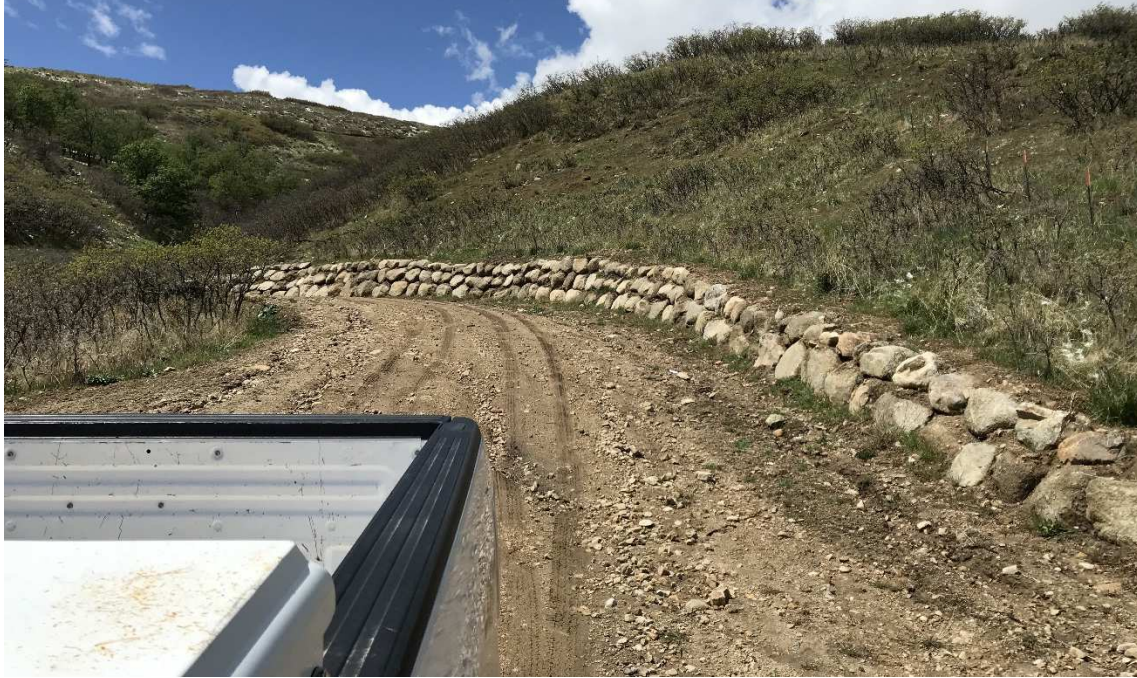
NON-COMPLIANT RETAINING WALL BUILT TO PROPOSED LOT 72
