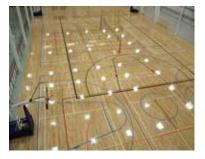
In addition to excellent uniformity, the VIP sandwich design results in limiting and dampening vibration.
