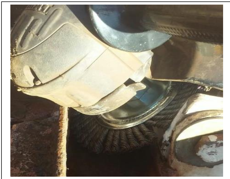
Gauge Pole Hatch showing the wire wheel being used
