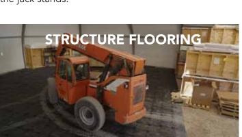
PortaFloor **MAX** was recently installed inside a Sprung® structure as a heavy duty reusable flooring system for inventory storage versus a gravel sub-base. The floor easily contoured to the structure's unique shape by including 6" wide cable-channeled **MAX** pieces that enabled a custom fit. **MAX** provided a firm stable surface for the rolling service doors. In structure installations, MAX can be installed inside the structure or extended beyond the sides for a clean and durable foundation.
